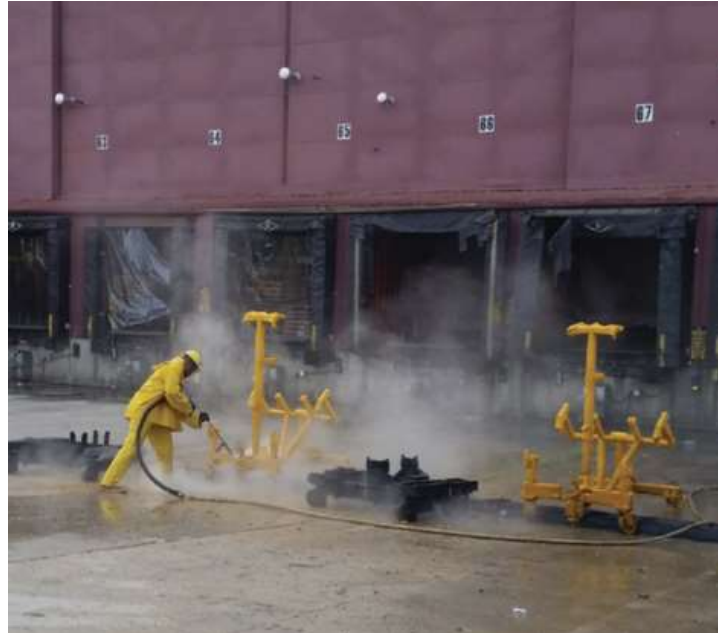
ABOVE: 40k PSI hydro-blasting of the paint carts
